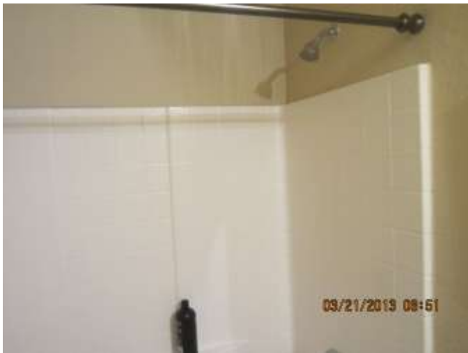
Picture #87 Shower Surround
