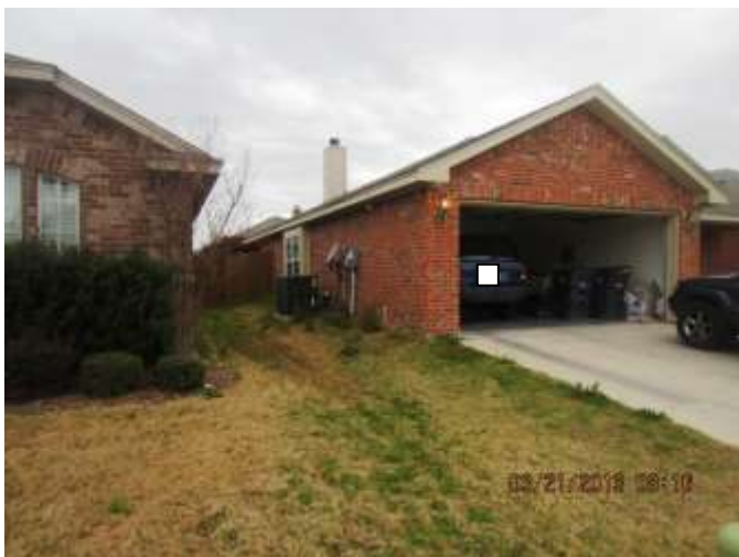
Picture #4 Side of House and Yard
