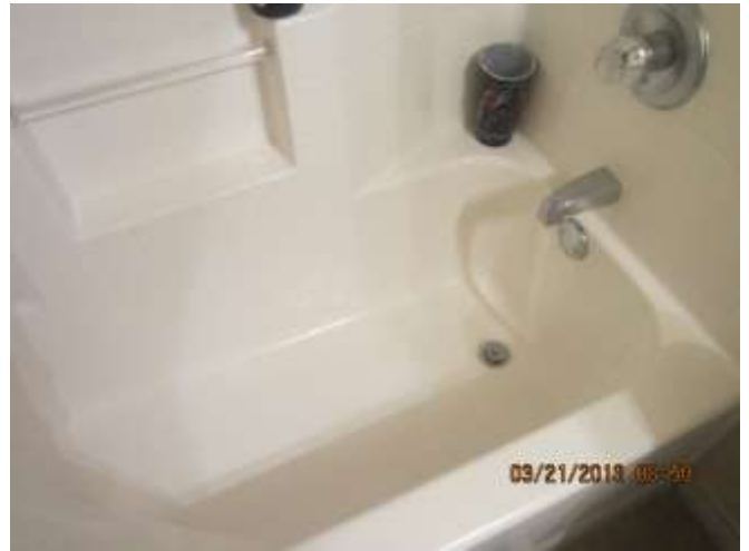
Picture # 86 Tub/Shower Surround
