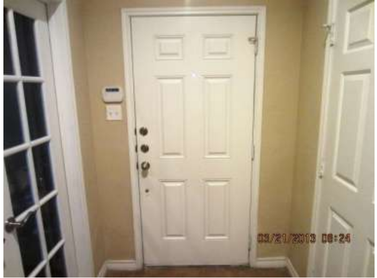
Picture # 20 Front Door including casing.
