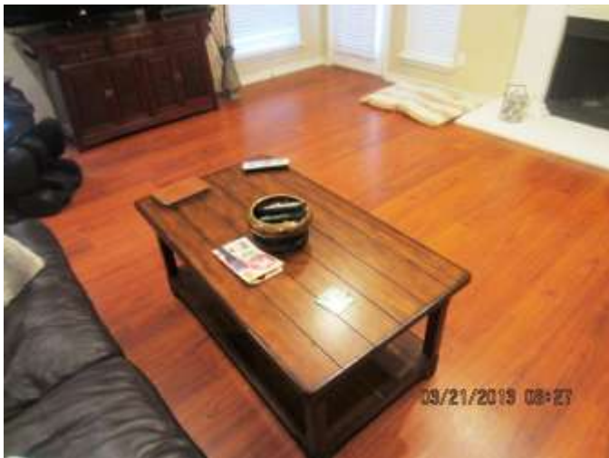
Picture #24 Living Room Floor
