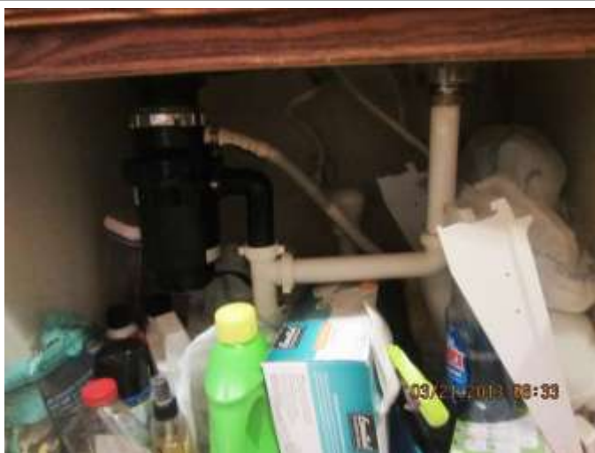
Picture #49 Cabinet Under Sink
