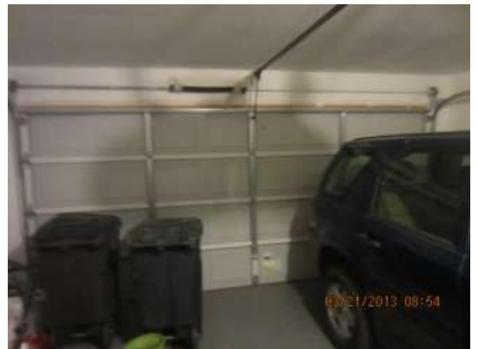
Picture #103 Garage Overhead Door
