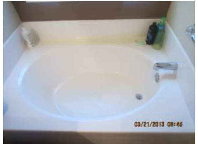
Picture # 64 Tub/Shower Surround
