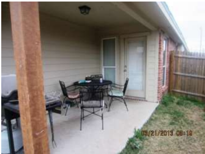
Picture #10 Rear Door and Porch
