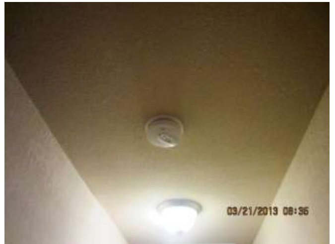
Picture #54 Hall Lighting/Ceiling
